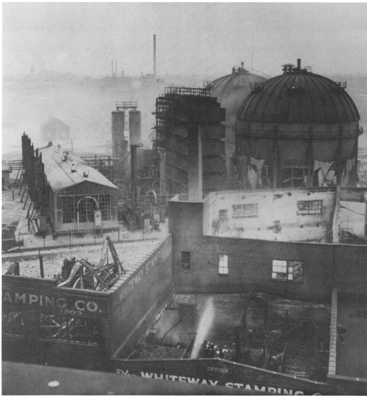
Figure 28.—General view of damage to LS & R plant, East Ohio Gas Co., looking east, showing spherical tanks 1 and 2 standing at the right and cooling tower with burned grids in the center and compressor building with broken window panes at left. Damaged building of the Whiteway Stamping Co., in foreground.
