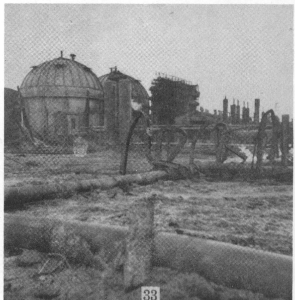
Figure 30.—Damage to east side of gas holder caused by heat from the fire.
